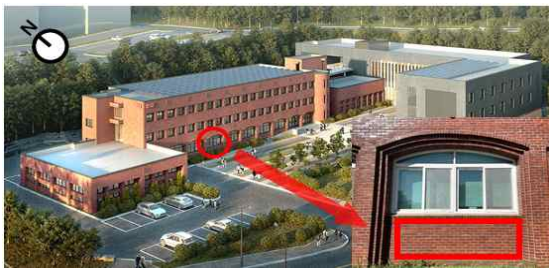
Fig 5. Measurement target building
